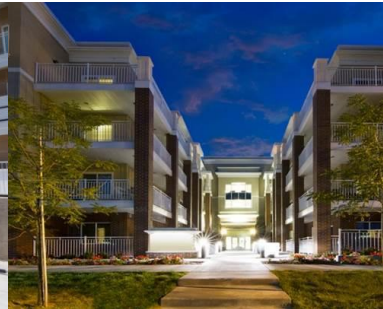
THE MERCER 556 EAST 300 SOUTH
