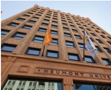
TOWER SUITES 143 SOUTH MAIN STREET
